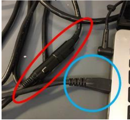
Fig. 6: Ethernet cable connections.
